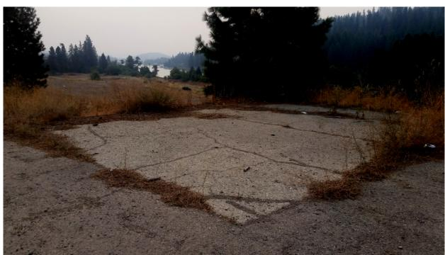
**Photo 10:** Looking southeast at the former aboveground storage tank area. This area was once used for refueling log trucks and included a 10,000 gallon diesel aboveground tank in secondary containment.
