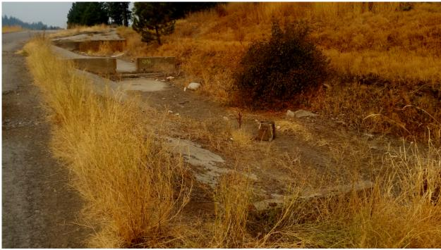
**Photo 18:** Looking west at the former weir system used for the partial concrete drainage area on the east portion of the site.
