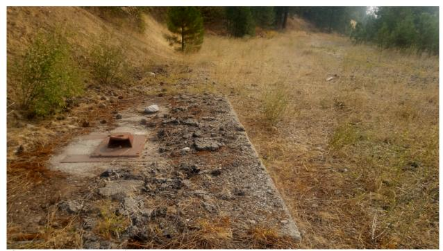
**Photo 17:** Looking east at a former winch anchor point along railroad ROW or a spur line. The device was used to move railcars.
