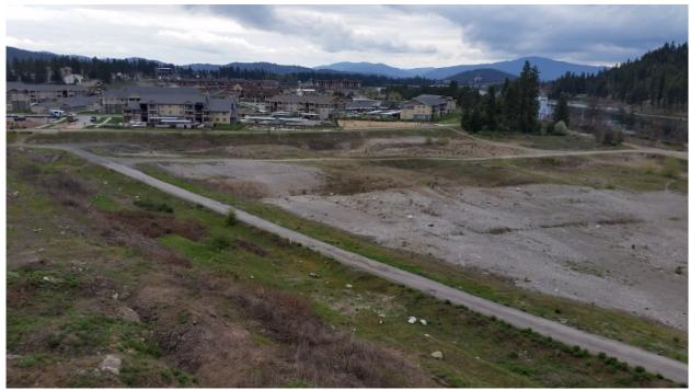
Photo 1: Looking southeast across the former lower log storage area on site (see Figure 3) and the former ROW of the NPRR. The area was scraped of top soil and debris, which was stockpiled on the northeast portion of the site. The Riverstone residential development and the North Idaho Centennial Trail are in the background.
