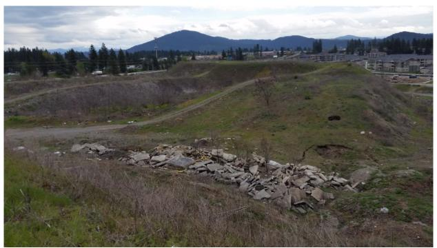
**Photo 8:** Panning right and looking easterly at the wood waste stockpile that also includes concrete debris. Subsidence is notable within the stockpile, which rises as much as 60 feet above surrounding landscape.
