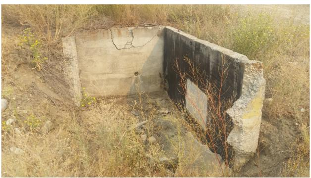
**Photo 14:** Looking at a former septic tank once located near the northern end of the sawmill building. Clay tile pipe was observed leading to this feature.
