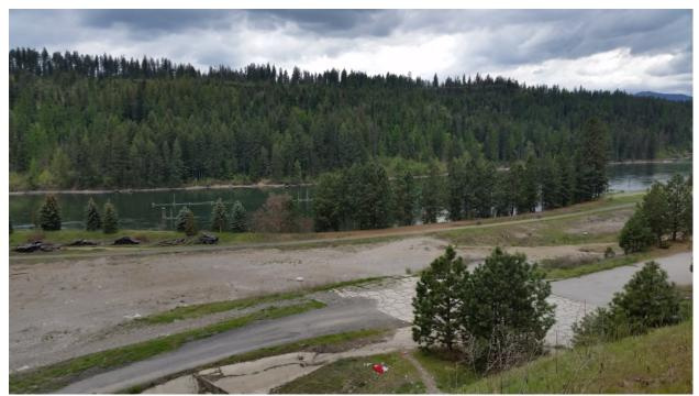
**Photo 3:** Panning right and looking southerly across the eastern central portion of the subject property. A partially concrete-lined drainage feature rests in the foreground. Water lines and utilities were observed behind trees on the lower right, but appeared disconnected and perhaps damaged.
